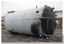
Photo 1 (above): Atmospheric storage tank following the fire.
